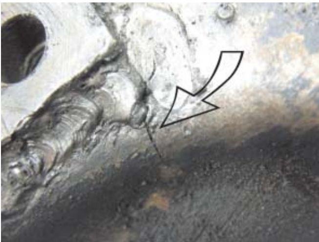
Figure 2. On the opposite front pad, a little wire brushing reveals a new crack starting to propagate. This is a significant and dangerous sign and should not be ignored.
