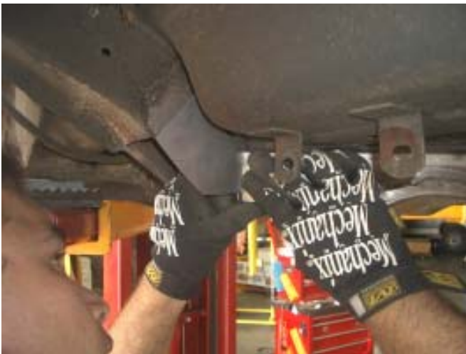
Figure 9. "Fitting" the side piece to the chassis.
