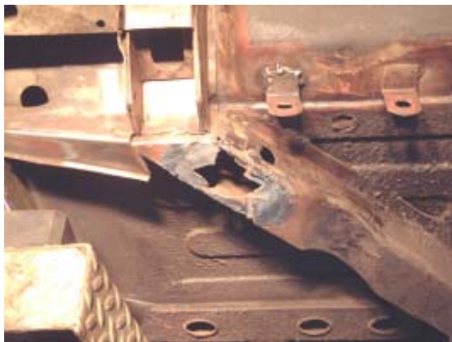
Figure 5. Here we have a typical Tiger frame that has "lost" the Weld-On Traction Master frame mount. The Weld-On mount is one of the weaker points and has often been torn off and re-welded to the X-member several times, resulting in this kind of damage. My recommendation is to switch to the Bolt-On design for the traction bars or eliminate them and use the Dan Walters developed Torque Arm (909 926-1572).
