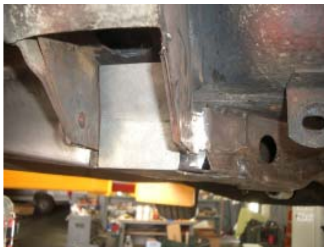
Figure 6. Here is the rectangular piece, bent and placed into position. Note that it is just below flush with the bottom of the chassis. You will be welding this edge, so you don't want it too high.
