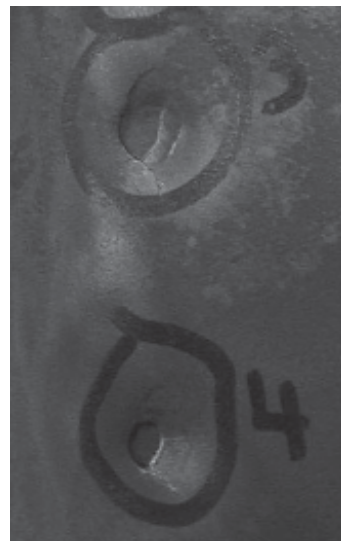
Figure 4. Here we have a closeup of the spot welds shown above. It is clear that the floor pan is failing and that the rear sub frame is pulling away.
